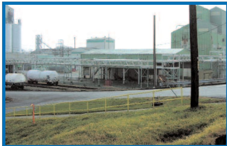
Two of the largest sources of mercury pollution are coal-fired power plants and mercury-cell chlorine factories.
